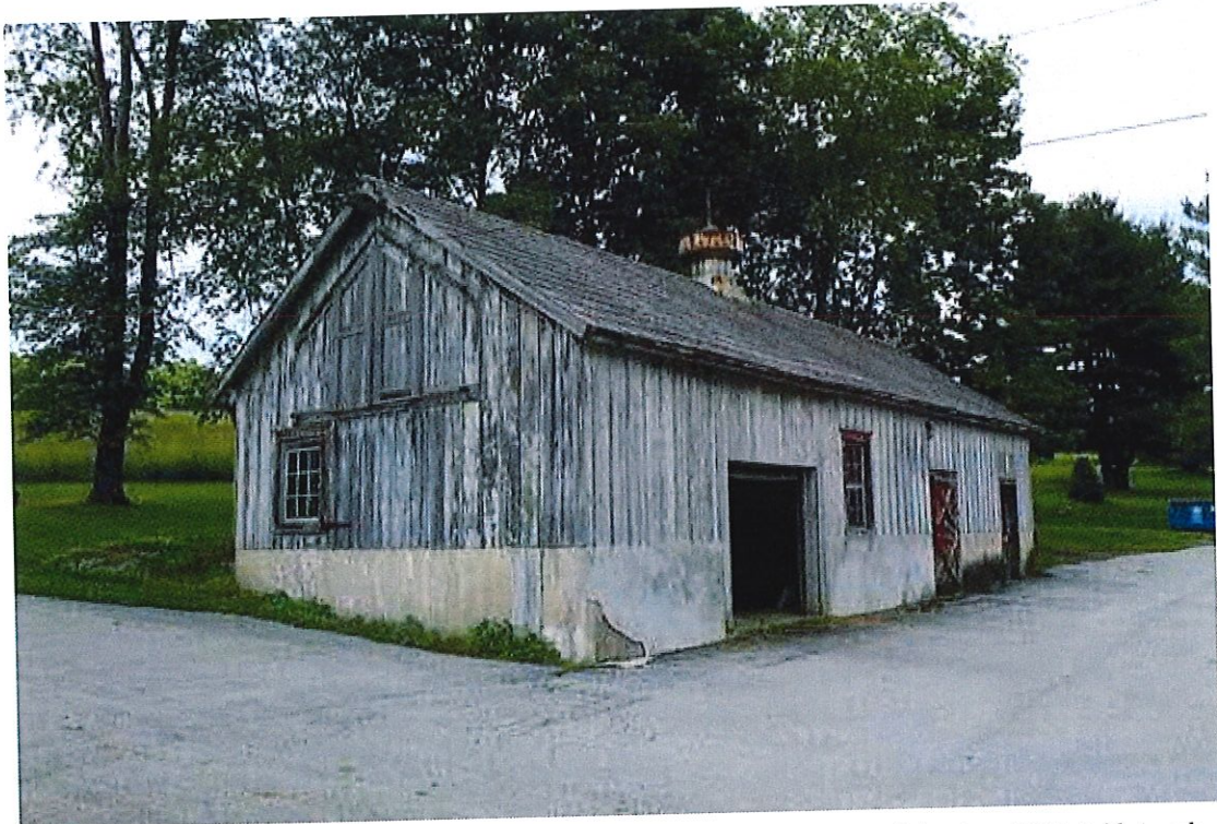
Photograph 12: View of the southeast (side) and northeast (front) elevations of the circa -1925 stable/workshop, facing west (June 2016).
