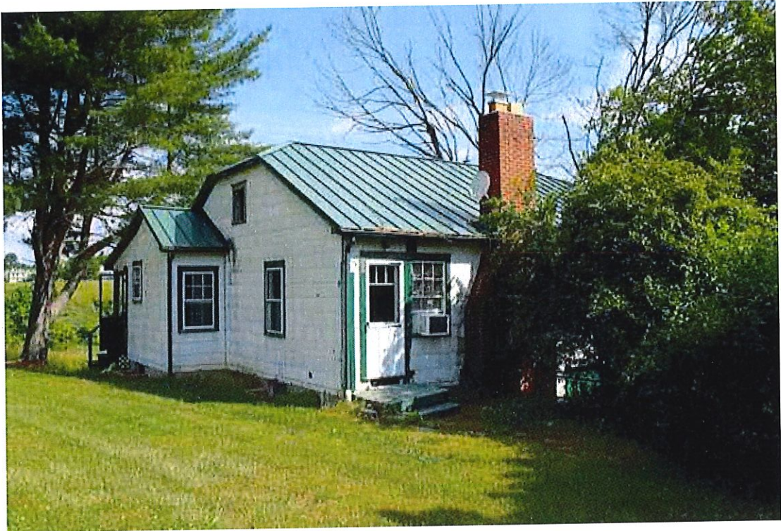
Photograph 7: View of the southwest (side) and southeast (front) elevations of the circa -1848 carriage house 1/ circa -1940 dwelling 2, facing north (June 2016).
