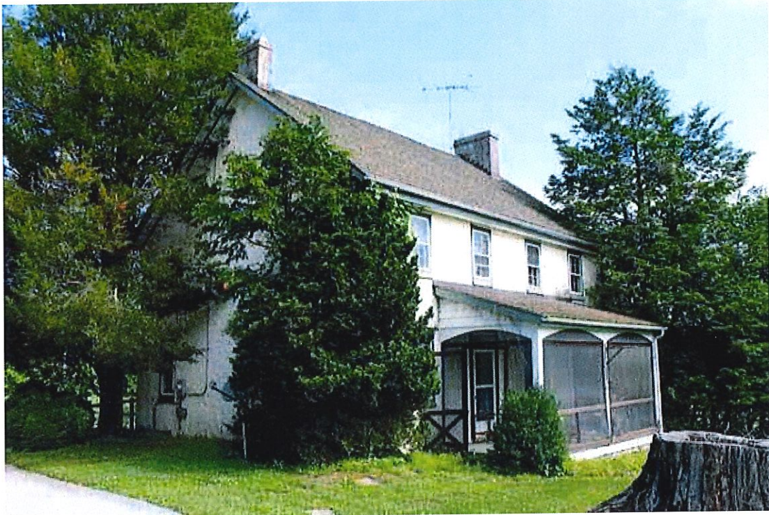
Photograph 1: View of the southwest (side) and southeast (façade) elevations of the circa -1848 dwelling 1, facing north (June 2016).
