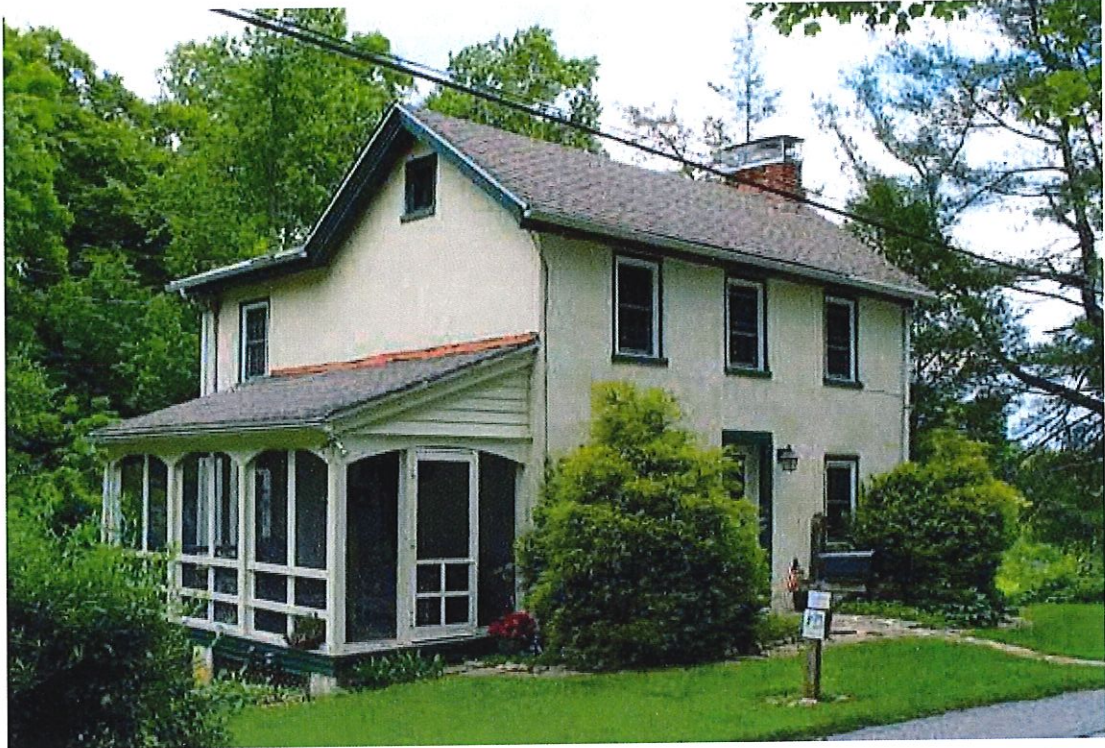
Photograph 37: View of the southwest (side) and southeast (front) elevations of the circa -1848 tenant house at 605 Norway Road, facing north. Note the one-story circa -1920 shed-roof porch addition and the two-story circa -1860 rear addition (June 2016).
