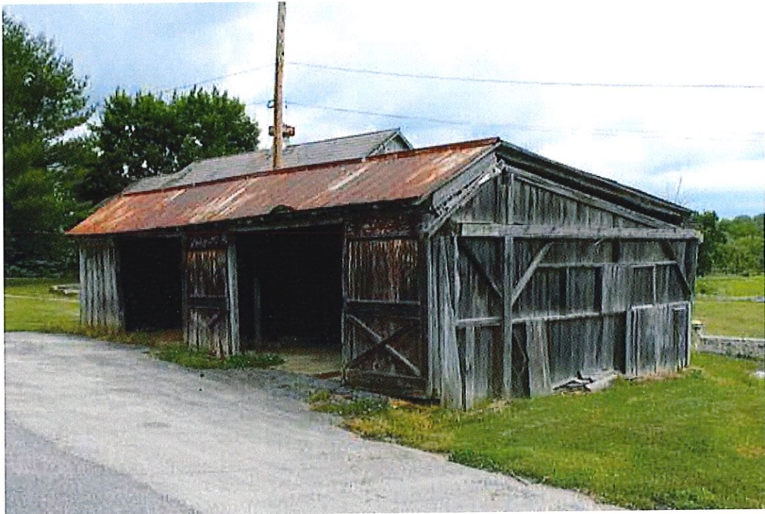
Photograph 17: View of the southwest (front) and southeast (side) elevations of the circa -1940 machine shed 2, facing north. Note the remnant framing from the earlier structure visible on the southeast elevation (June 2016).
