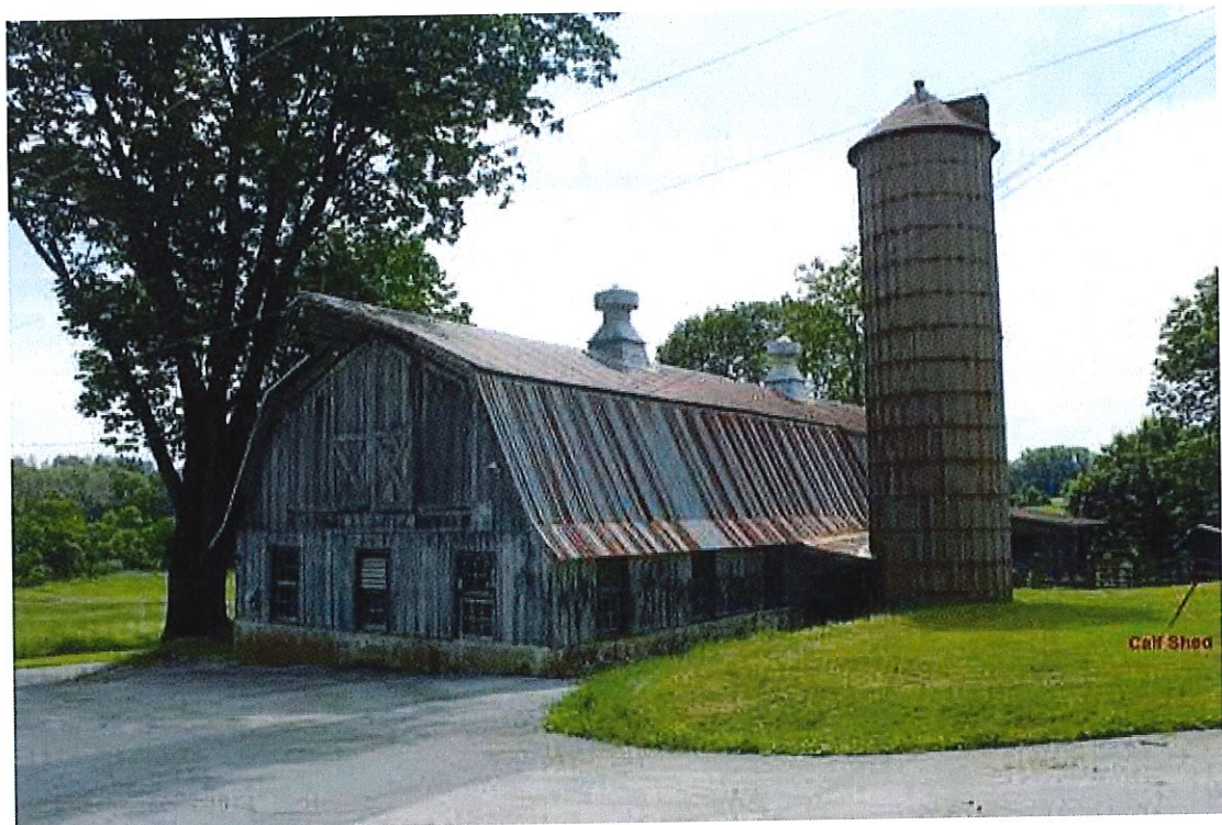
Photograph 14: View of the northwest and southwest elevations of the circa -1925 cow barn 1 and silo, facing east. Note the circa -2013 calf shed (far right; June 2016).
