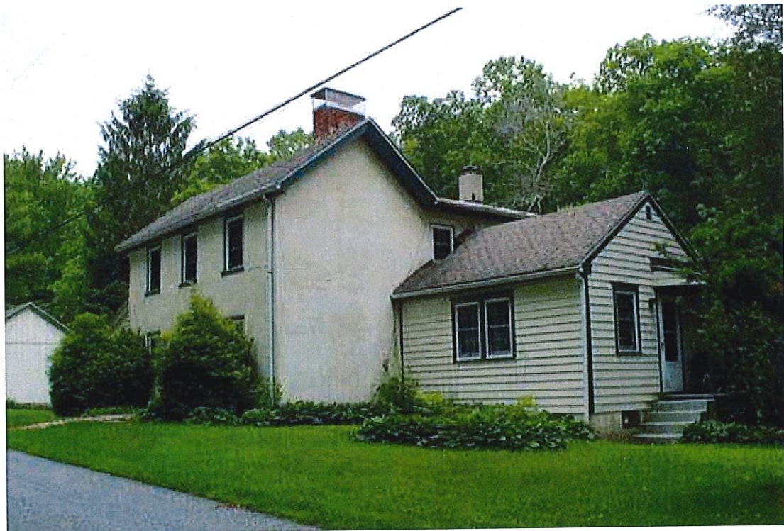
Photograph 38: View of the southeast (front) and northeast (side) elevations of the circa -1848 tenant house, facing west. Note the circa -1880 summer kitchen addition (at right; June 2016).
