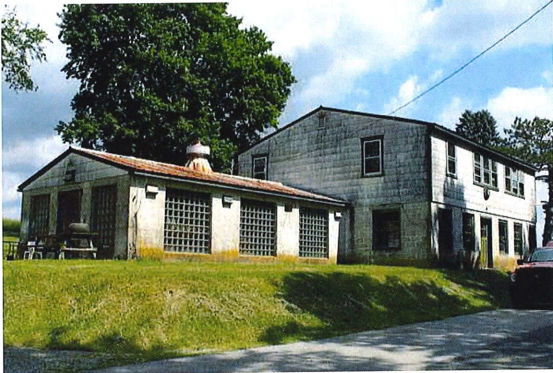
Photograph 19: View of the southwest (side) and southeast (front) elevations of the circa -1940 turkey house, facing north. The one-story south addition (left) and two-story turkey house core (right) are visible in this photograph (June 2016).
