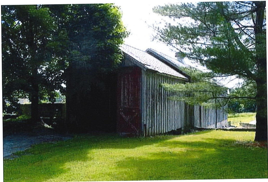
Photograph 8: View of the northwest (front) and southwest (side) elevations of the circa -1925 machine shed, facing east. The hay barn is to the rear of the machine shed (June 2016).
