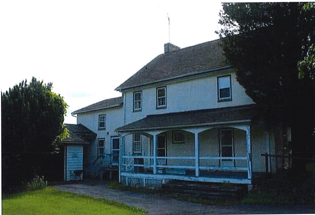
Photograph 3: View of the northwest (rear) elevation of the circa -1848 dwelling 1, facing northeast. Note the garage (far left; June 2016).
