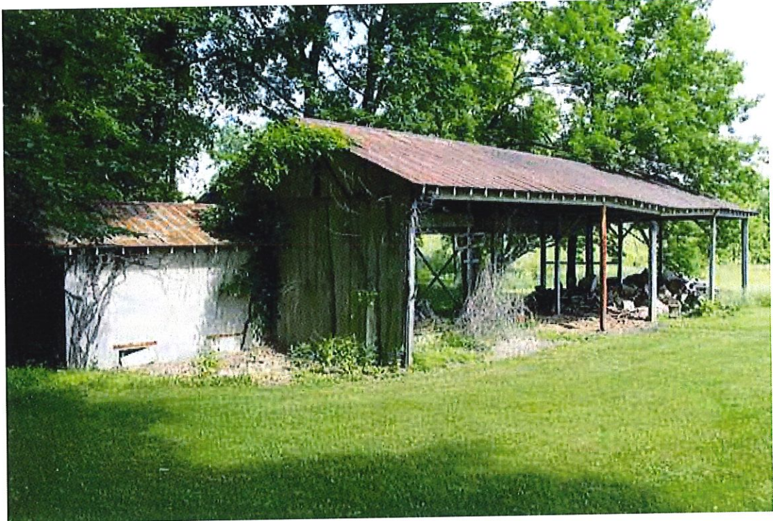
Photograph 29: View of the south (side) and east (front) elevations of the circa -1950 equipment shed, facing northwest (June 2016).
