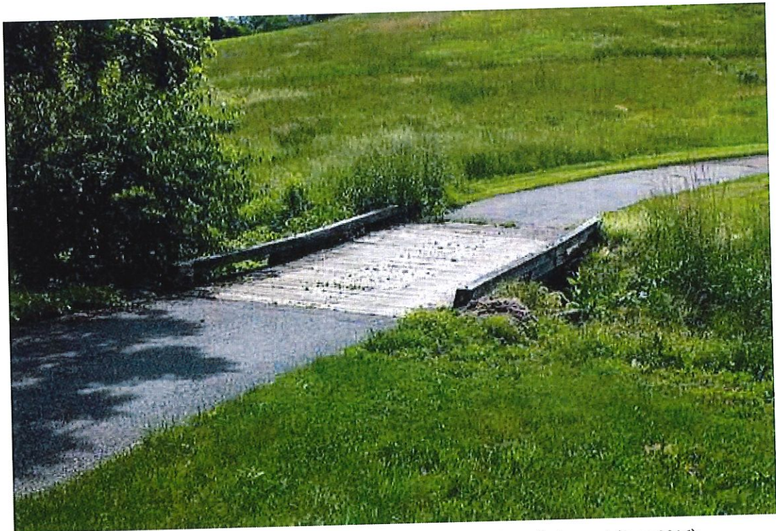
Photograph 16: View of the farm lane bridge crossing over Barrows Run, facing east (June 2016).
