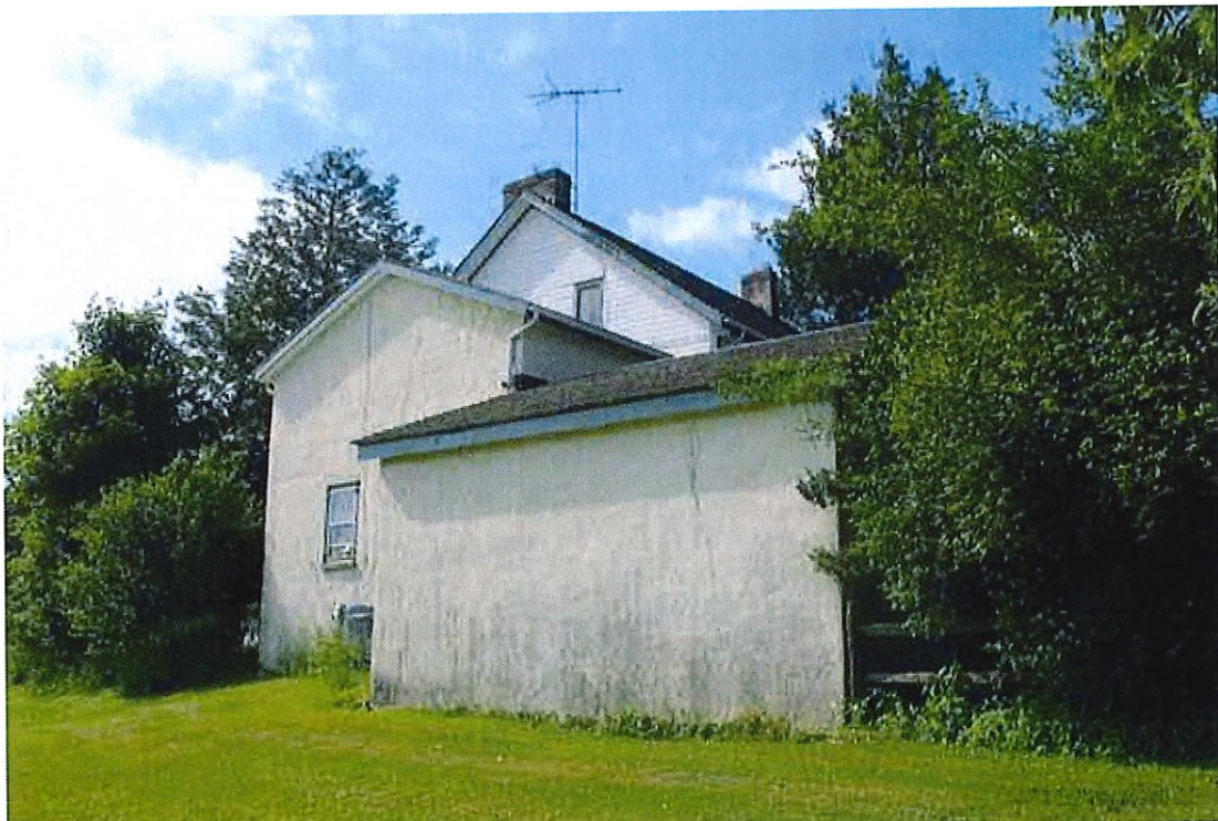
Photograph 2: View of the northeast (side) and northwest (rear) elevations of the circa -1848 dwelling 1 and circa -1848 outbuilding/ circa -1940 garage 1, facing south. The outbuilding's (foreground) northwest and northeast walls are of stone construction, while the opposite walls are wood frame construction. Based on its location to the dwelling, it is likely that this building was a wash house or a summer kitchen, but it was fully converted into a garage ca. 1940. Note the northeast end of the main block of the house (background). This wall is of wood frame construction while the other three walls of the main block of the house are all built of stone (June 2016).
