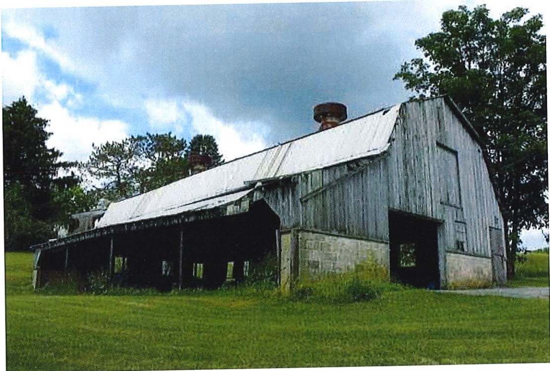
Photograph 31: View of the southeast and northeast elevations of the circa -1955 cow barn 2, facing southwest (June 2016).
