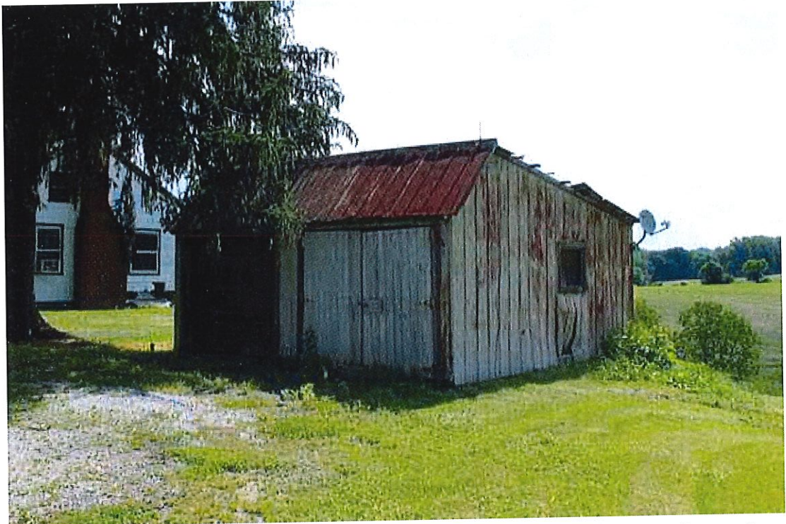
Photograph 27: View of the northwest (front) and southwest (side) elevations of the circa -1940 garage 2, facing east (June 2016).
