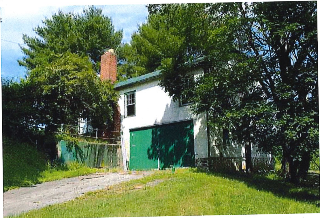
Photograph 5: View of the southeast (front) and northeast (side) elevations of the circa -1848 carriage house / circa -1940 dwelling 2, facing west. Note the stone foundation at the northern end of the building (right). The first story of this building was built for use as a carriage house. Ca. 1940, the second story apartment was added (June 2016).
