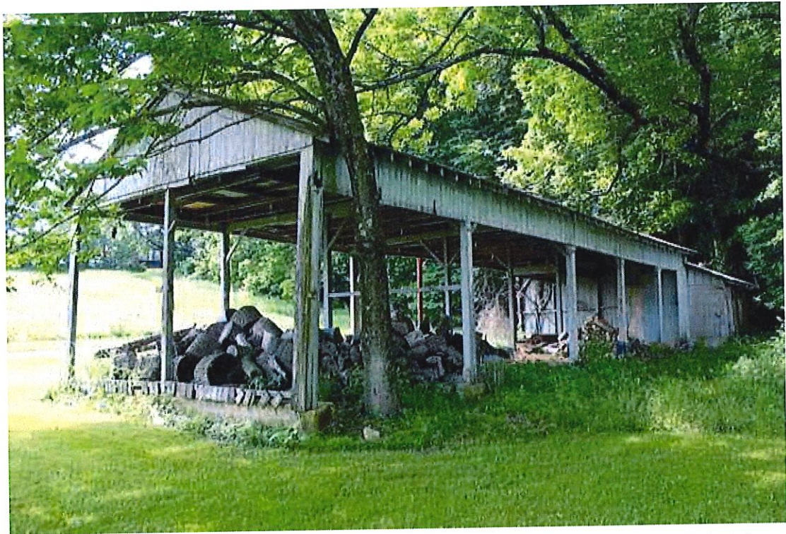
Photograph 30: View of the north (side) and west (rear) elevations of the circa -1950 equipment shed, facing southeast (June 2016).
