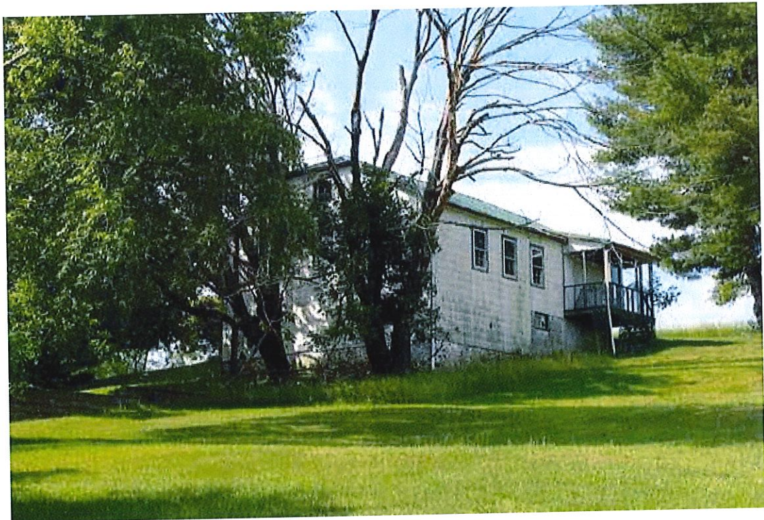
Photograph 6: View of the northeast (side) and northwest (rear) elevations of circa -1848 carriage house 1/ circa -1940 dwelling 2, facing south. Note the change in foundation material approximately half way along the northwest elevation showing the circa -1940 second-story apartment addition (June 2016).
