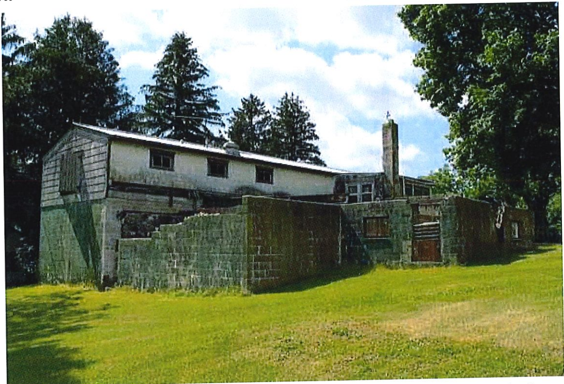
Photograph 21: View of the northeast (side) and northwest (rear) elevations of the circa -1940 turkey house, facing south. The ruins of the circa -1955 addition are clearly visible in the foreground. The concrete block chimney marks the location of the rear elevation of the turkey house core (June 2016).
