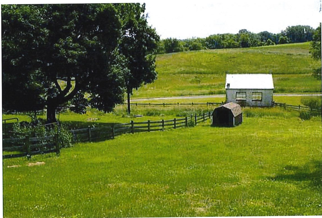
Photograph 34: View of the northwest (front) elevation of the circa -2003 shed and the northwest (rear) elevation of circa -1955 garage 3 showing the fenced cow runs and pasture, facing east. Barrows Run flows through the farmstead at the far end of the pasture, demonstrated in this photograph by the tall grass (June 2016).
