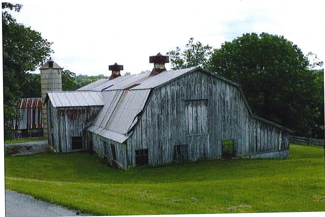
Photograph 32: View of the northwest and southwest elevations of the circa -1955 cow barn 2, facing northeast (June 2016).
