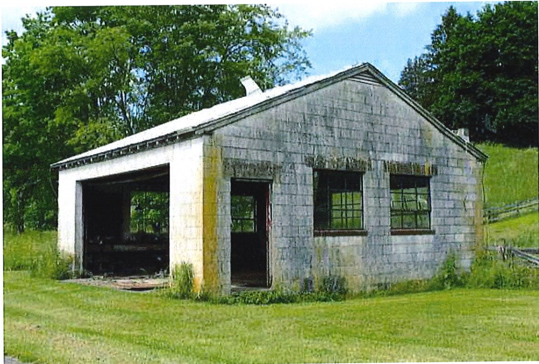
Photograph 33: View of the southeast (front) and northeast (side) elevations of the circa -1955 garage 3, facing southwest (June 2016).
