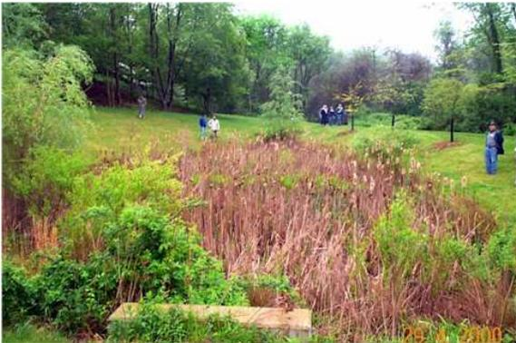
Wet Ponds/Retention Basins are stormwater basins that include a substantial permanent pool for water quality treatment and additional capacity above the permanent pool for temporary runoff storage.
